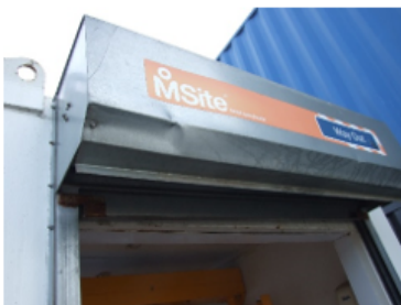
Dent to Roller Shutter
