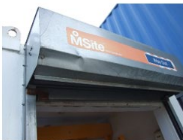
Dent to Roller Shutter
