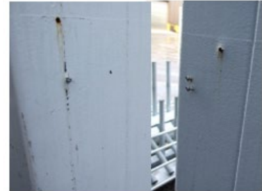
Bolt holes inc screws and bolts attached
