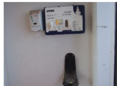
Customer equipment left in unit – removal, repair and holes to fill
